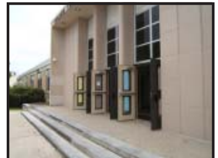
Memorial Middle School Entry will become accessible under American with Disabilities Act
